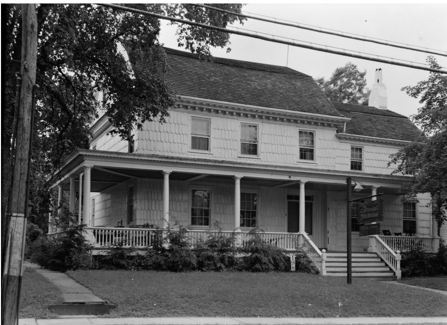
Photo 7. Front elevation (HABS NJ, 13-MAT, 1), 1936 (Nathaniel R. Ewan photograph).
