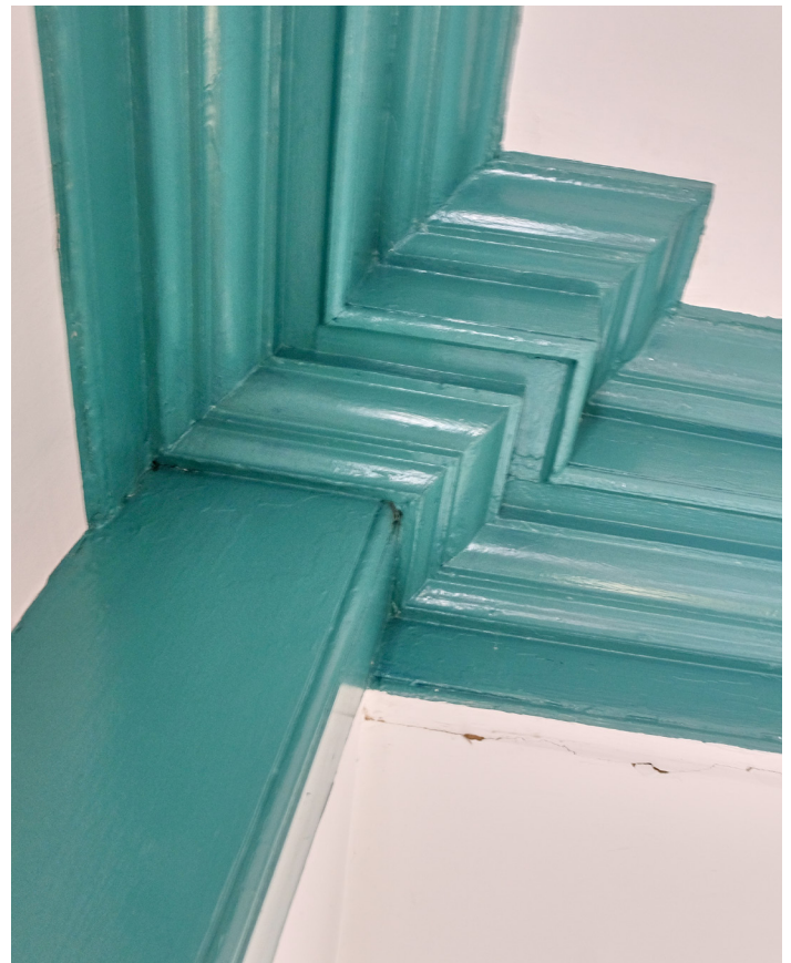
Photo 2. View of a full-section corner post and the crown moulding which wraps around the posts, 2025 (C. Cielo photograph).
