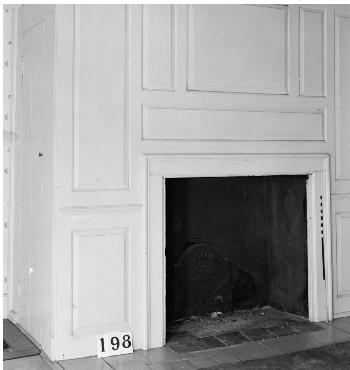
Photo 5. Second floor front chamber (HABS NJ, 13-MAT, 1), 1936 (Nathaniel R. Ewan photograph).
