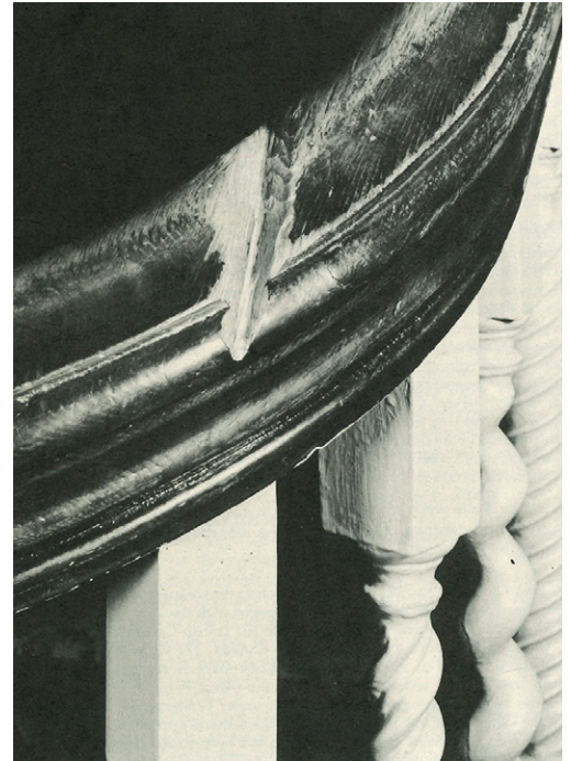
Figure 3. Detail showing the wedge of wood chopped out of the Schuyler house railing (Schuyler Mansion HSR, 1977).
