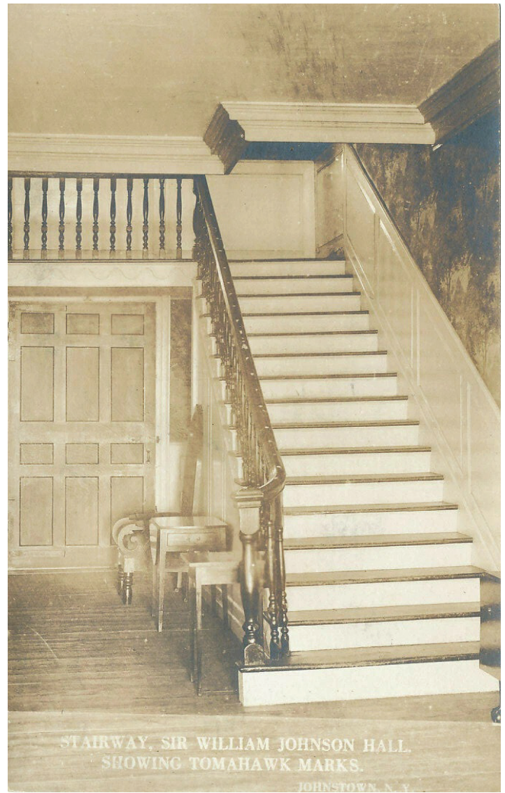
Figure 1. Johnson Hall stairway, ca. 1908 (Private collection). The damage to the railing appears as white spots, the cuts reflecting glancing light.
