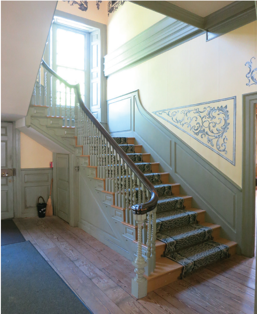
Figure 2. Main staircase at the Schuyler Mansion, Albany (Author photo, May 2019). The cut in the hand rail is located at the point where it begins to turn toward the newel.
