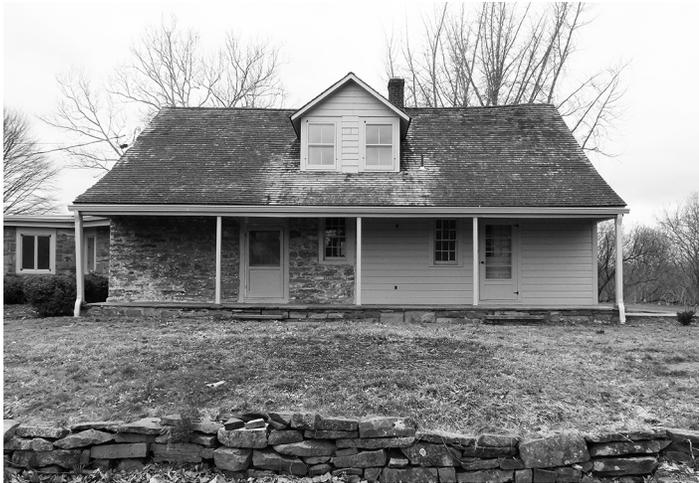
Fig. 6 – Benjamin Freer House, Bontecoe. An early timber-framed one room house c.1715 with a stone addition c.1730.
