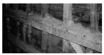
View of recycled hay-barrack post at north end wall in bent in three-bay three-aisle barn at the Oliver homestead. Note holes at corner of post that functioned in raising and lowering of adjustable roof in former hay barrack. Round pole studs appear above and below the post.
