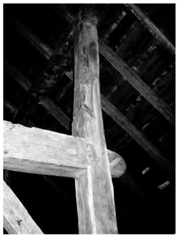
View of H-frame post that was later spliced circa 1830 in four-bay threeaisle classic barn at the Oliver homestead. Note hewn rafters in common rafter system in roof.
