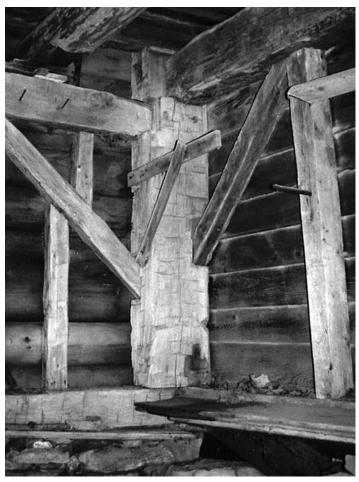
View of the substantially sized oak corner post in one of the one-aisle barns at the Oliver homestead. In upper left corner large round pole joists are seen to support floor above.
