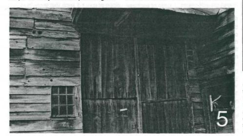
Seen are original wooden hinged single height doors at last interior H-frame in Bogart U-barn in Marbletown, Ulster County, New York. Doors lead into the last bay, full of dirt. At sides of both door posts are remnant horizontal sheathing.
