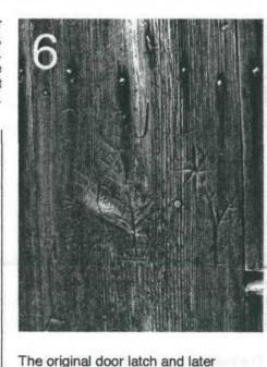
included "pull-open" mechanism is intact. Each door side was originally of two halves - an upper and lower. Lower door halves are unique in that they are double sheathed. Very unusual folk like carvings were rendered on one of the lower door halves. (Photo 6) In addition, extremely rare original pentice arms survive which actually appear as poles that emanate from the first inner anchorbeam which then extends over the end wall anchorbeam and beyond close to 4 feet.
