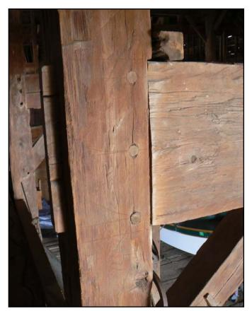
Photo 5. Detail of one of the anchor beam ends, showing scribe marks and small tenon projection (Ned Pratt).
