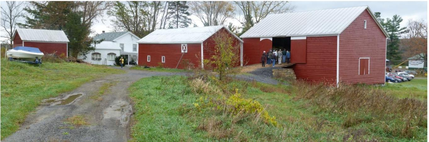
This barn was built partly into the side of the hill, suggesting it and the ramp may have been built at the same time. It is also a three bay barn, and the Upper level seemed remarkably similar to the first barn we saw. However, here all the smaller members and the uprights are sawn, but with an up and down saw, suggesting this is earlier than the Saddlemire barn.
